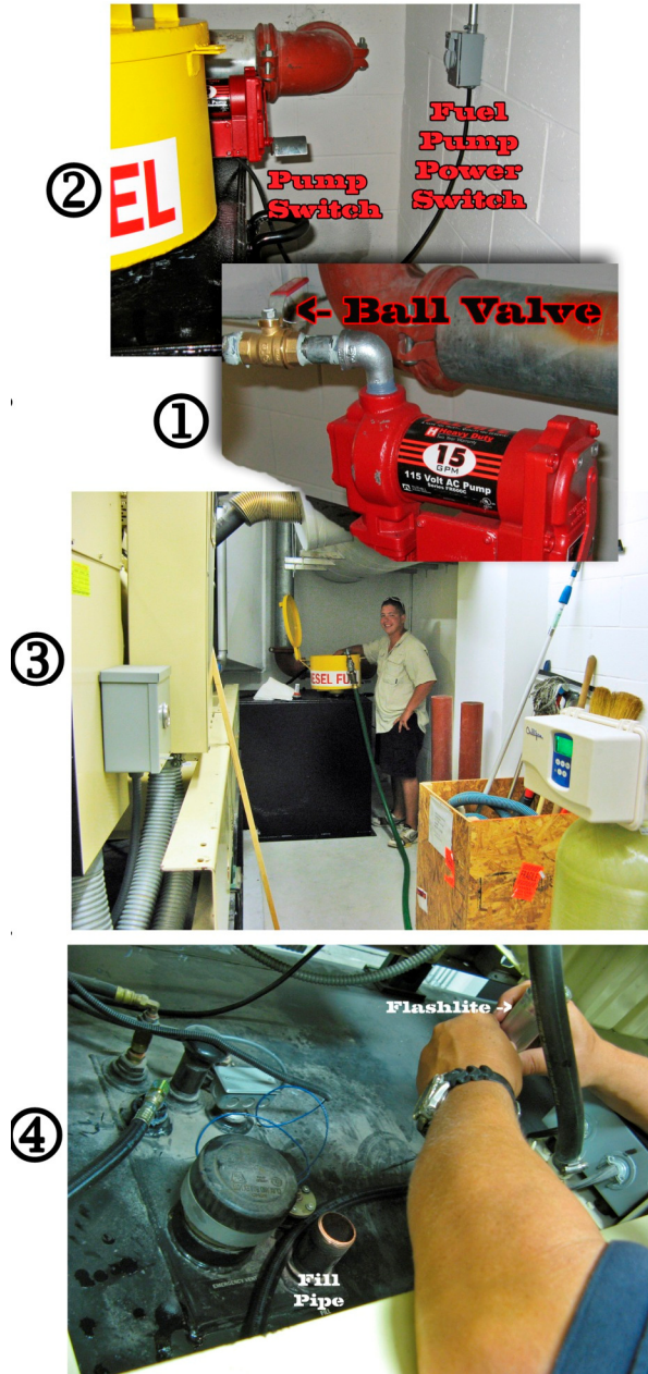
Figure 2.3.9 Fuel Tank Filling Details
