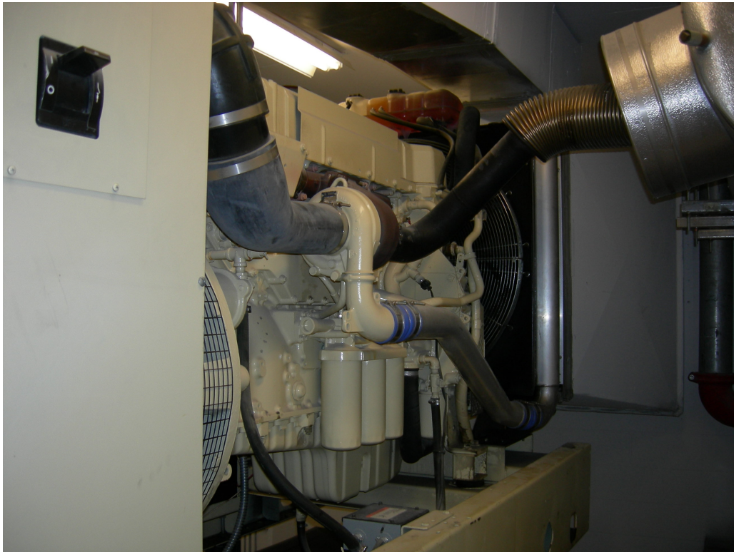
Figure 2.3.3 Savoy Motor Generator Set-Left Side View
